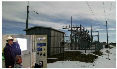
When inside a substation, SCADA webpages for that local substation can be viewed when attached to the Orion RTU. SCADA pages from other substations can also be viewed. Photo is from a Colorado substation.
