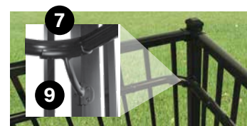
Inside Corner Mount & 90° Elbow Detail
