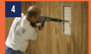
4 Drill hole in basement wall.
