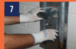
Install wall plate & tighten system.
