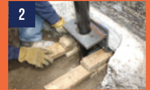
2 Install the bracket.
