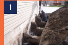
1 Expose the footing.
