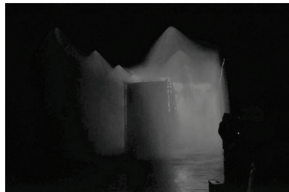
Figure 1 FOGTEC Deluge System
