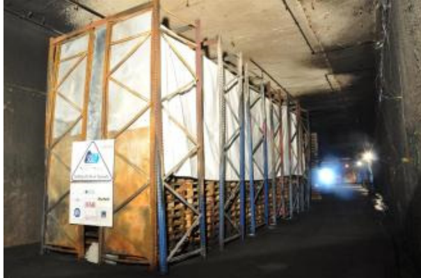
Figure 7: SOLIT Truck Fire Load with Cover
