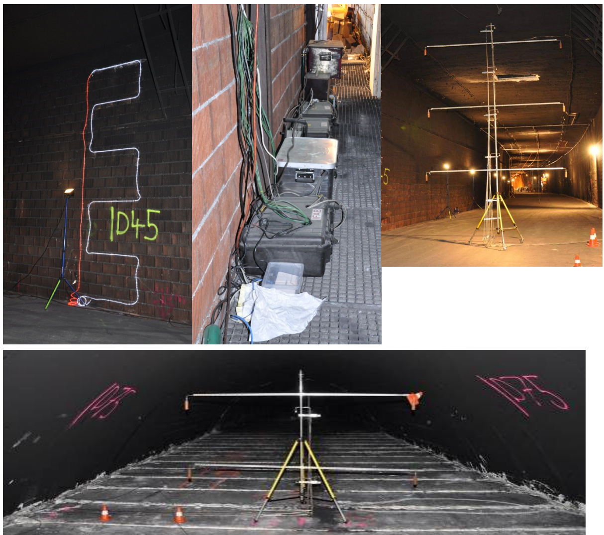
Figure 5: Various measurement equipment in the test tunnel
