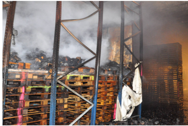
Figure 12. Example of undamaged target after a fire test [31]
