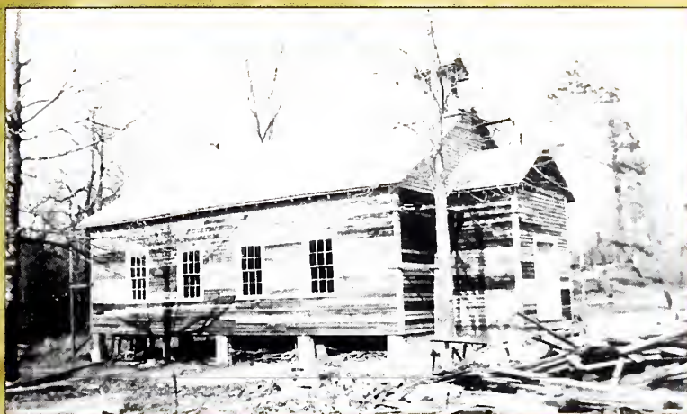
SIXTH AND CURRENT MEETING HOUSE Pictured Under Construction, 1942
